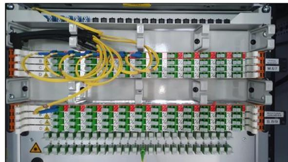
Figure 9: Fiber patches to connect CU/DUs with RUs
