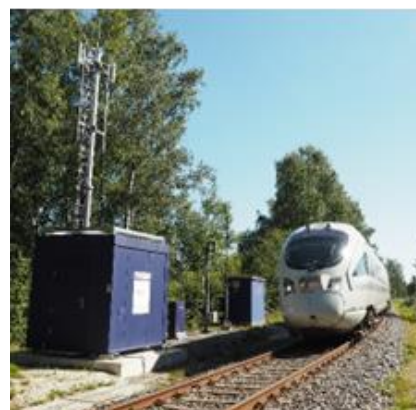
Figure 29: DB's experimental ICE train "advanced TrainLab" in the 5GRAIL Testbed Germany
