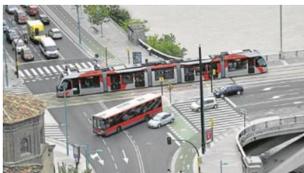
Figure 9: Intersection between tram and road traffic in the city of Zaragoza (Spain)
