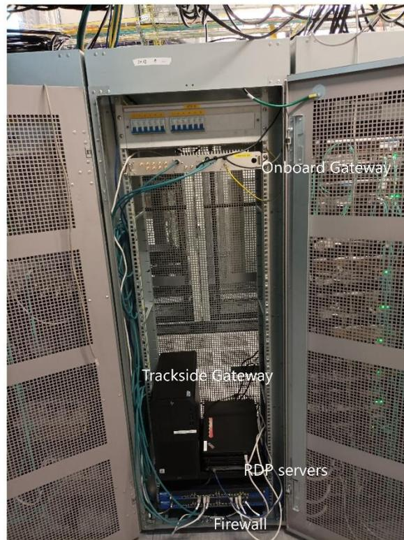
Figure 21: Hardware installation of gateways
